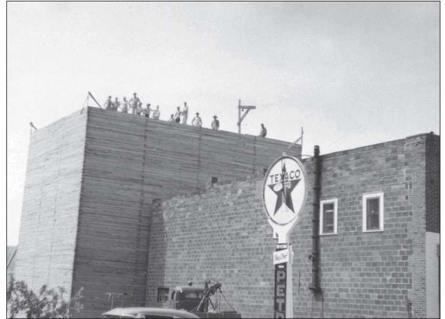
Grain Elevator under construction - 1955
